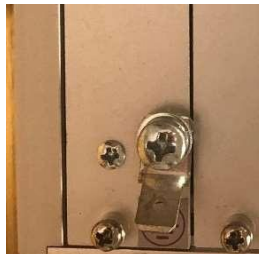
Picture 3-5-1-1 Earth connection point of the device at the Power supply module
